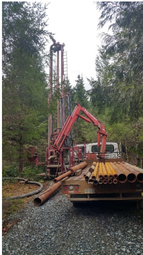
Photo A2: Drillwell setup on site with D12 Dual Air-Rotary Rig
