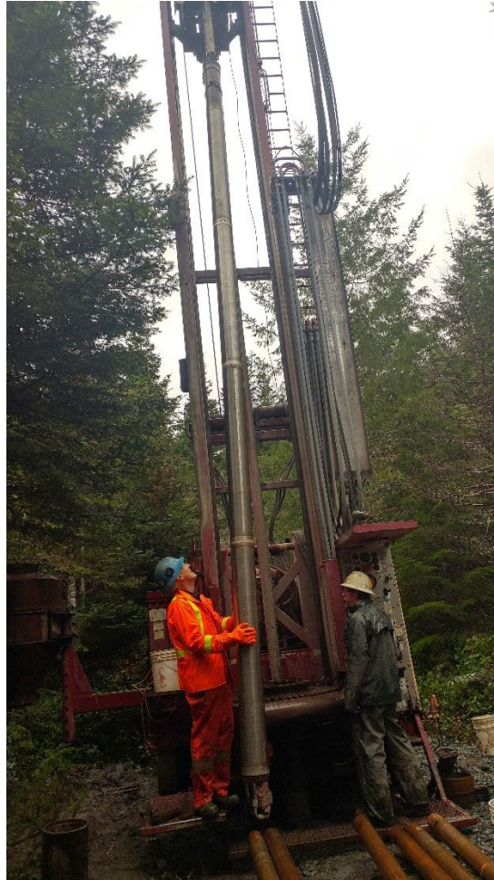
Photo A5: Installing 15' (4.57 m) of 30-slot stainless steel wire wrap screen
