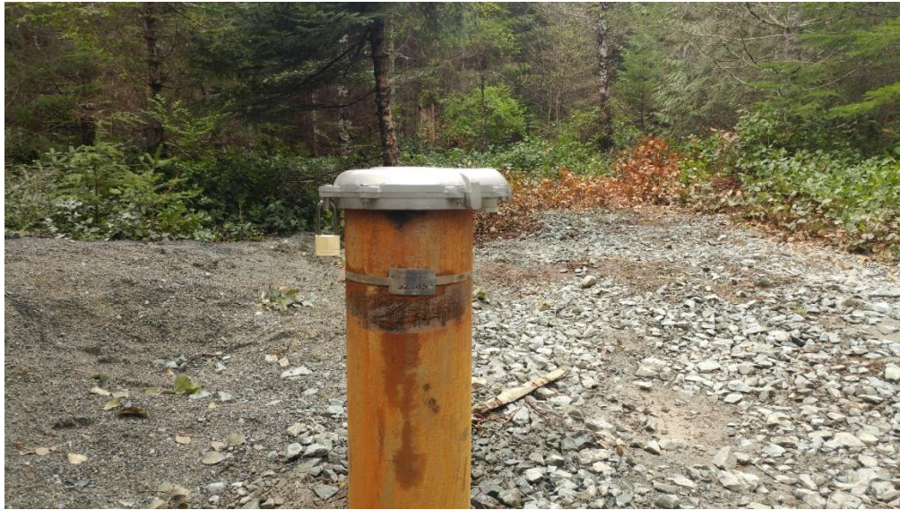
Photo A9: Completed well and well cap; ID Plate Number 52145
