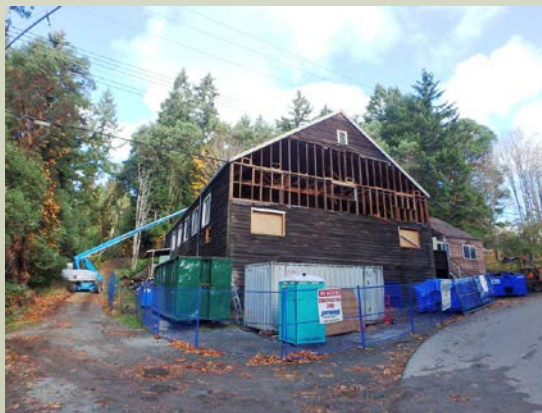
Siding being removed
