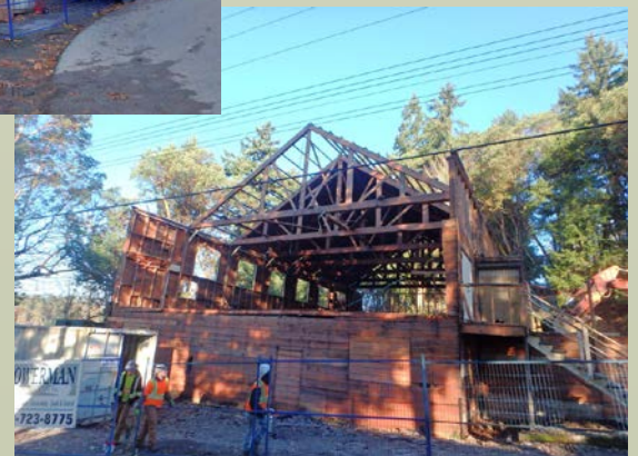
Siding being removed
