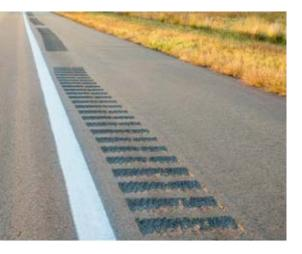
The BC Active Transportation Design Guide describes rumble strips as milled sections of the pavement along a roadway that provides feedback to motorists through noise and vibrations in the steering wheel, notifying them when they have deviated from the travel lane into the shoulder. Rumble strips are intended to clearly delignate the shoulder area and ensure the additional road width does not lead to higher vehicle operating speeds.
