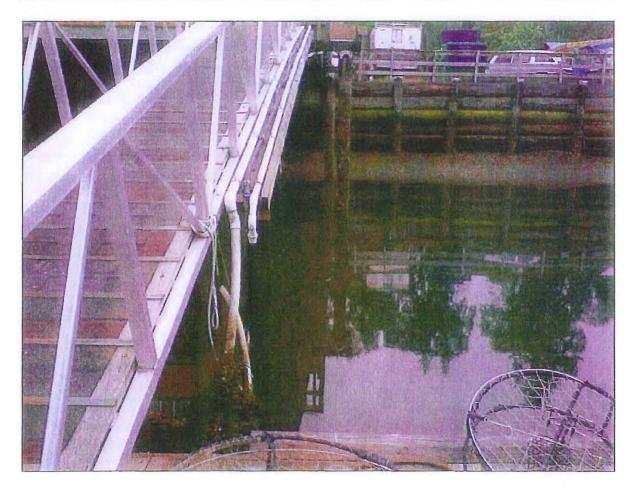
• The Force Main Continues under the dock where it is believed to tie into the gravity sewer servicing a number of buildings including a restaurant before entering the CVRD sanitary sewer.
