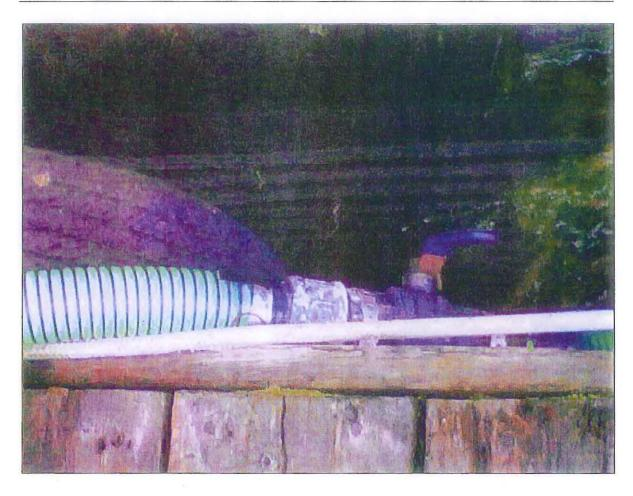
The hose is routed through the wharf system occasionally submerged into the water
