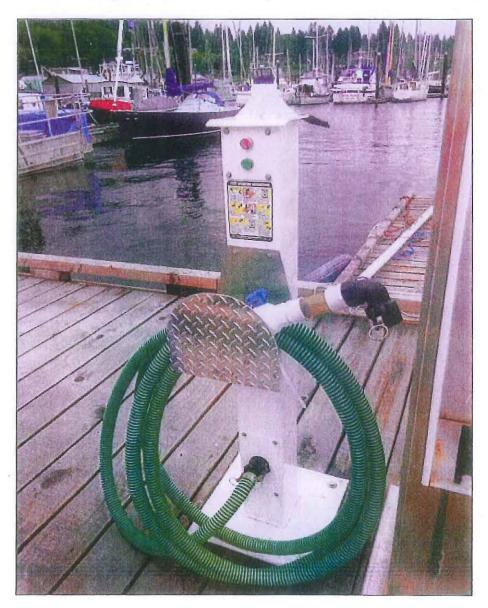
The sewage is transferred from the Boat Sanitation Dump through butt fused HDPE 50mm(High Density Polyethylene) pipe located just beneath the decking by the suction side of a pump located at the bottom of the ramp in a secure aluminum box.
