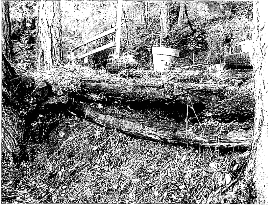
Photograph 3. View of old log cribbing containing the fill slope of the driveway.
